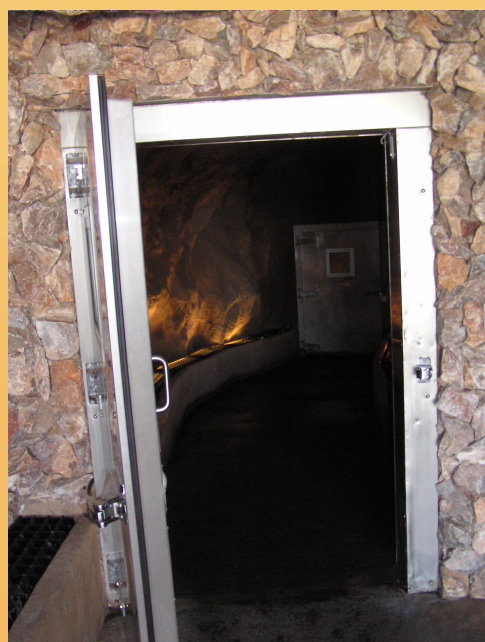
Visitors pass through several pairs of freezer doors. These airlock-like chambers limit mixing of outside and cave air.
